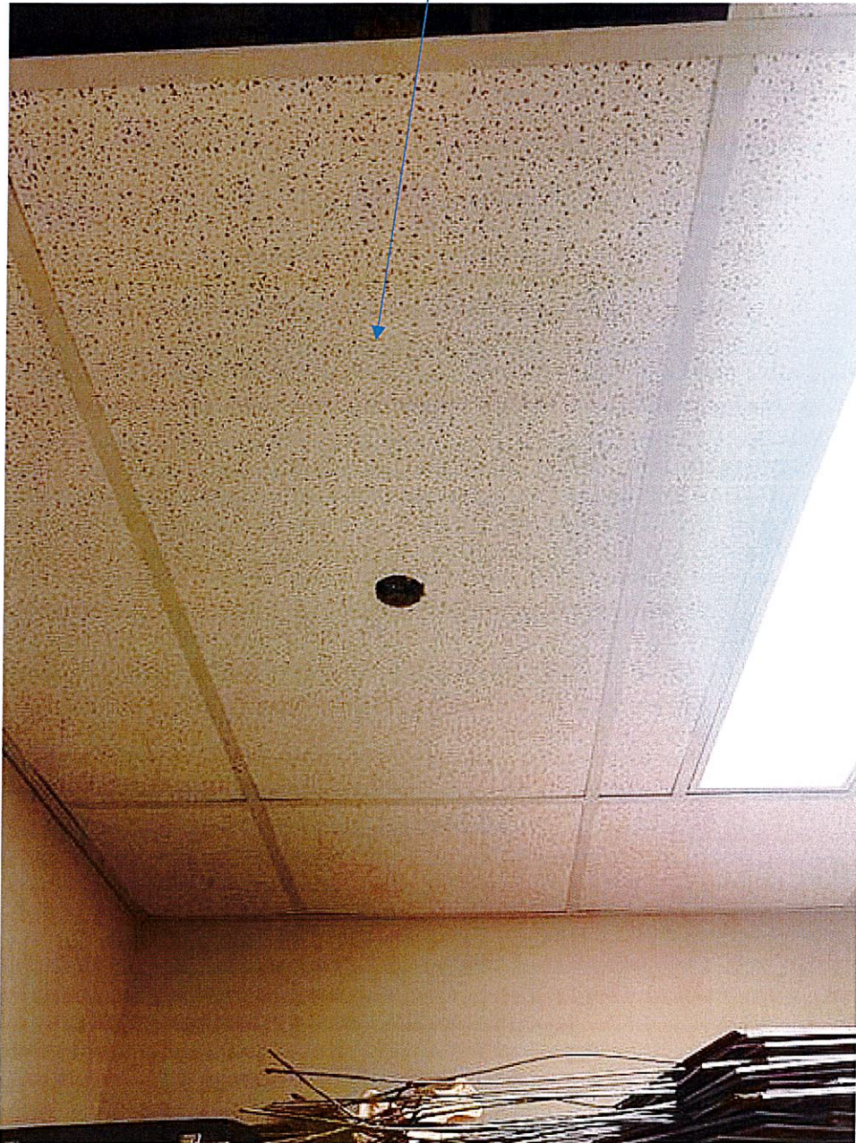
Room 238 – 2x4 ceiling tile – pins – non-Acm
